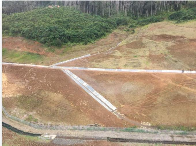
**Figure 4.4: Replacing Geofabric Ditch Liners at Komo with Concrete**
